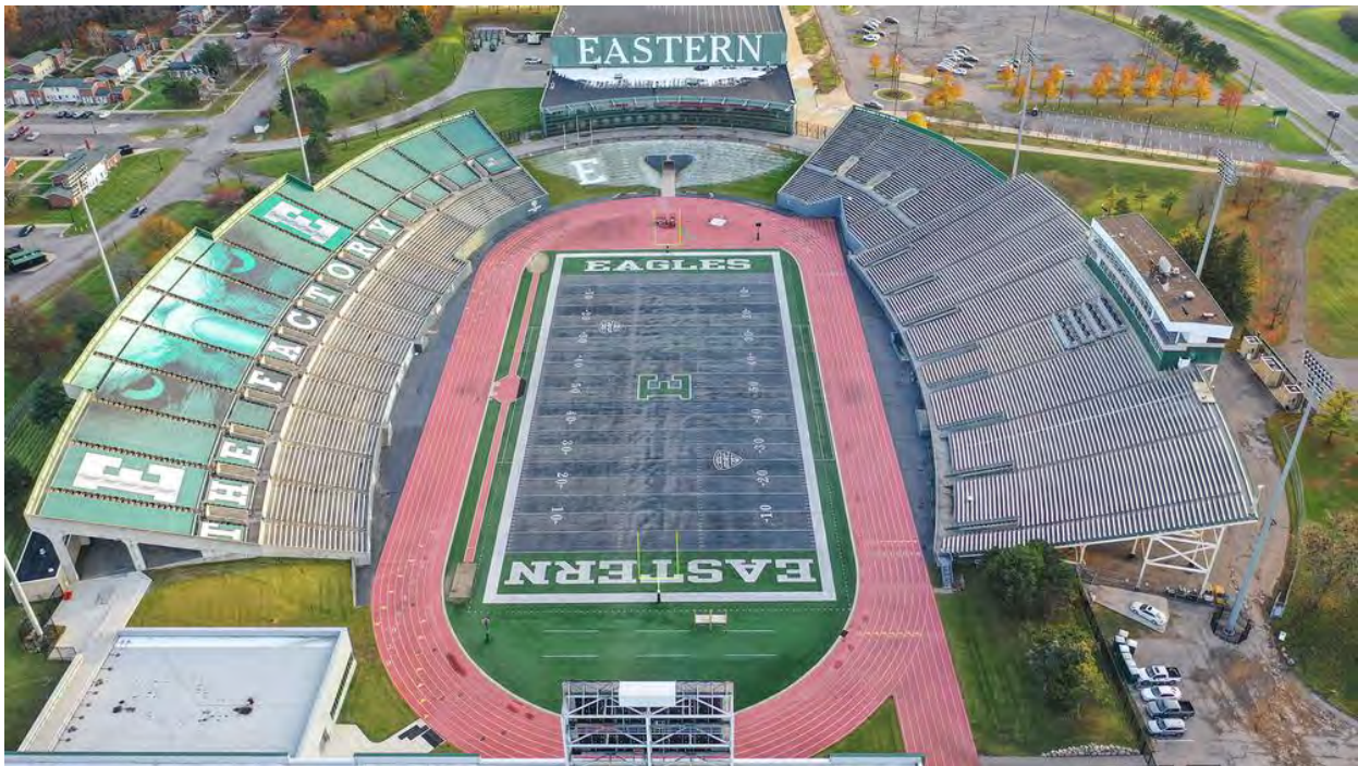
Figure 3-8: Aerial view of Rynearson Stadium
